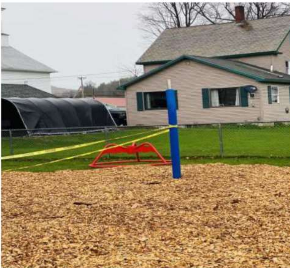
Caption 7: The circular maypole will be installed once the cement is hardened, 10/31/2020.
